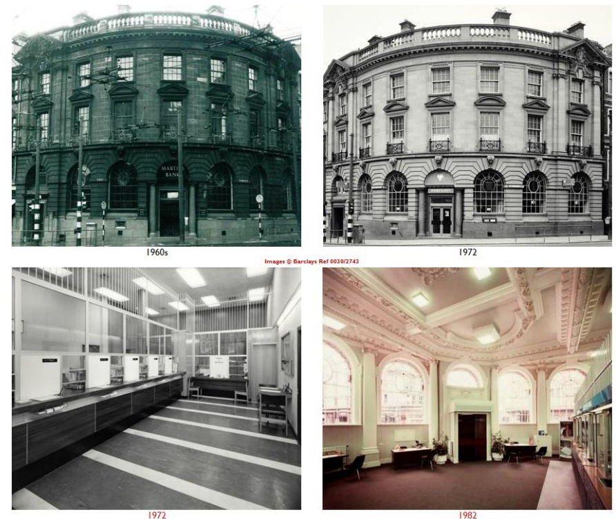
Figure 8 Historic Images of the bank from clockwise top left 1960s’, 1972, Banking Hall pictured in 1982 and 1972 counter (Martins Bank Archive Collection)
