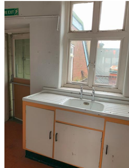
Figure 24 Fourth floor rear modern access stair and existing kitchen area in No 8 Fowler Street.
