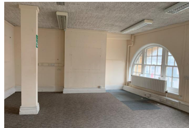
Figure 17 Change to room layout to north of the building, with evidence of wall removal, dropped ceilings and modern lighting/radiators and pipework.
