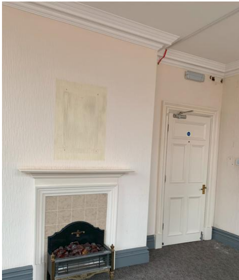
Figure 16 Historic panelled door, coving, skirting and fireplace surrounds (fire and tiling a later alteration).
