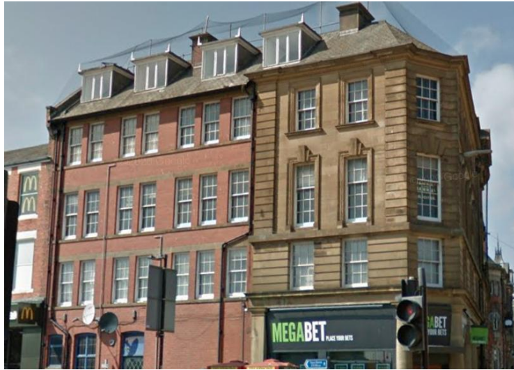
Figure 9 View of 4-6 Fowler Street from the south showing contrasting styling
