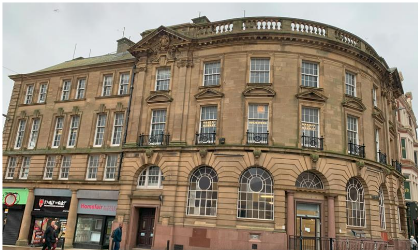
Figure 1 Application property viewed from the corner of King Street and Fowler Street.
