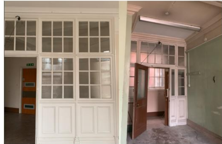
Figure 18 Historic panelled screens to be retained in redevelopment
