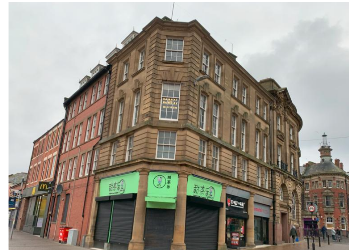
Figure 3 View of the property 4-8 Fowler Street from corner of Keppel Street and Fowler Street, ground floor commercial units excluded from site boundary.
