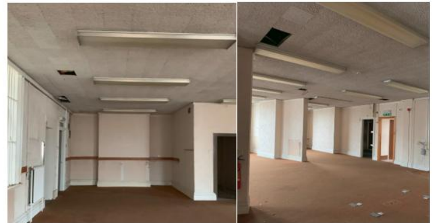
Figure 22 Third floor showing changes to plan form and dropped ceiling, vault shown to left image open plan space to right.
